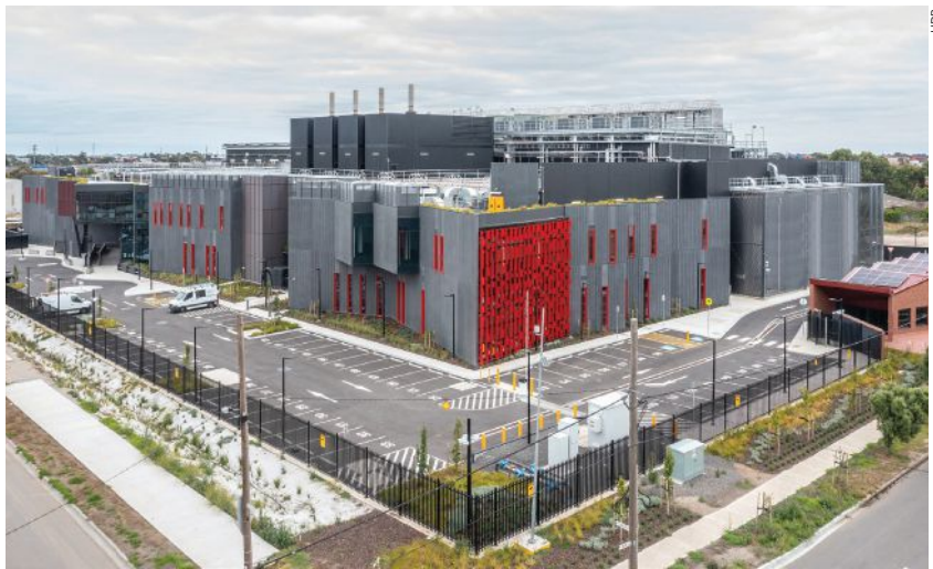
^ The 645,834-sf, 80-MW NEXDC Merlot 3 data center, located in the suburb of Melbourne, Australia, designed by HDR, operates as a colocation facility for retail, enterprise, and hyperscale customers. To respect its neighbors, the building is set back 20 meters, and that zone features a community café along a tree-lined perimeter that transitions the site from residential to industrial.
