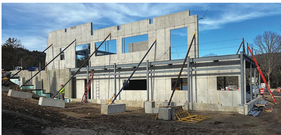
The designers for the DEEP project designed a thermal mass wall utilizing concrete made with post-consumer ground-glass pozzolan cement to optimize the site's solar orientation all year round. The Trombe wall provides passive heating and cooling and improves natural ventilation.
